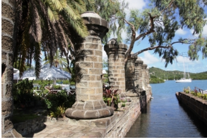
Stone columns at Nelson's Dockyard used to support a huge sail loft.
